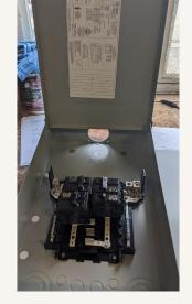
The old wiring to the hoist and shop has been replaced and new breaker box is in place. This was a much needed repair for a smooth operation of the hoist.
